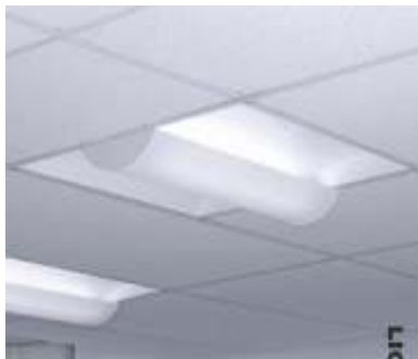
New ceiling tiles & light fixtures:
