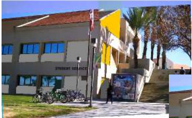
Paint existing stucco areas :
