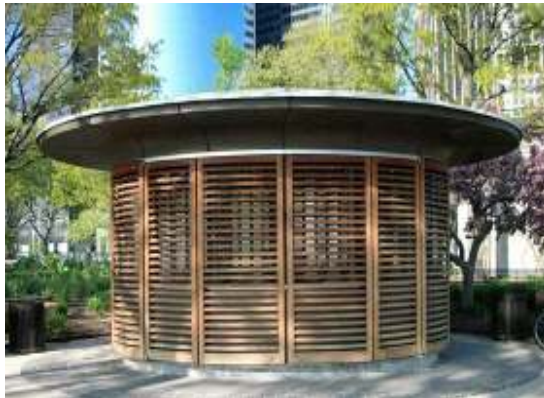
Semi Permanent Structure example:
