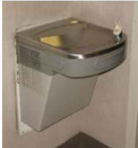
Existing drinking Fountains.
